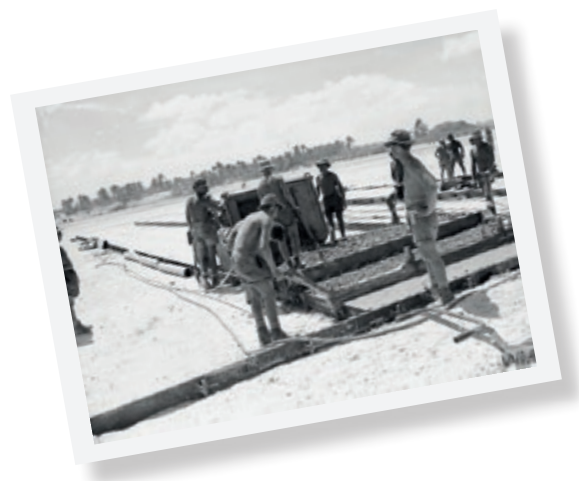
Wikimedia Commons / Royal Engineers construct the airfield runway on Christmas Island
