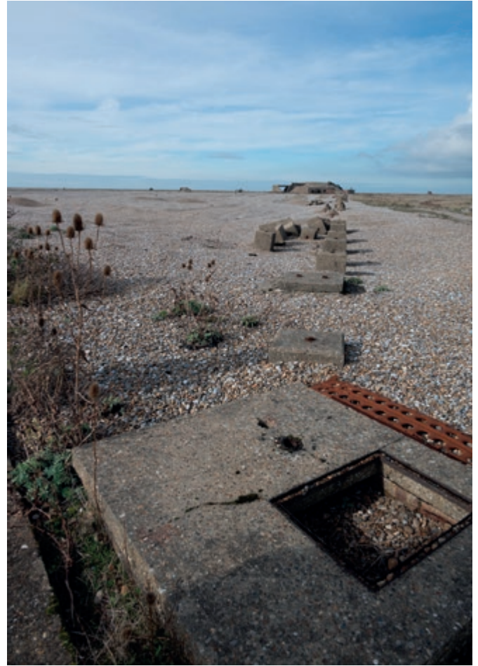
A line of decaying bases that held communications lines
