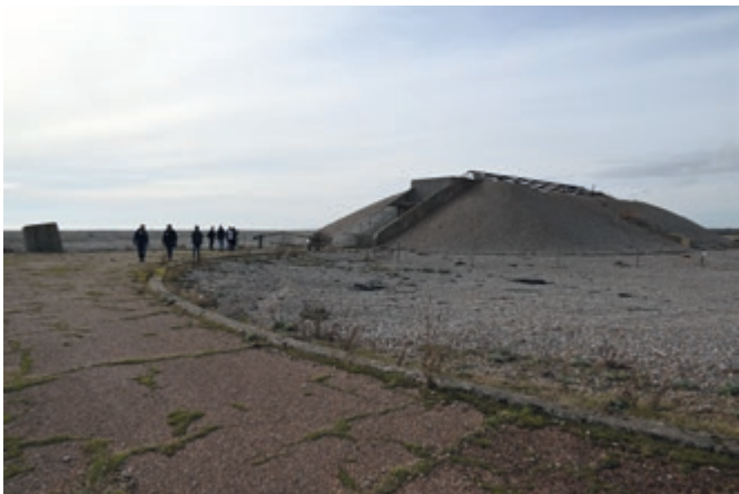
Laboratory 1 - tested six atomic weapons test cells constructed by AWRE Aldermaston
