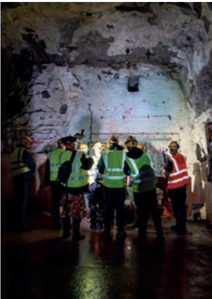
Viewing a opening through a bricked up tunnel section
