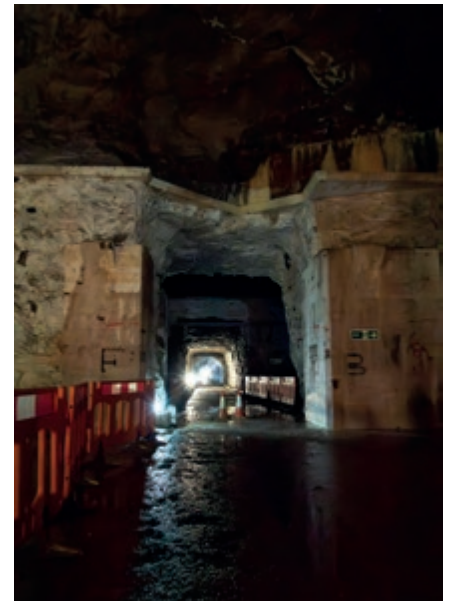
Looking back to the entrance
