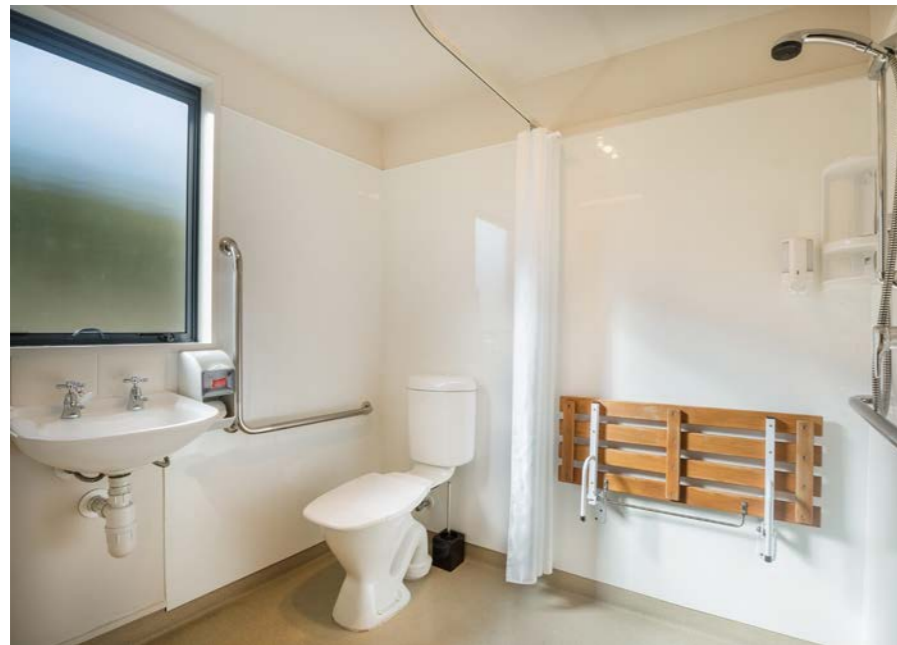
The beneficiary's downstairs toilet and coal house was turned into a wetroom.
